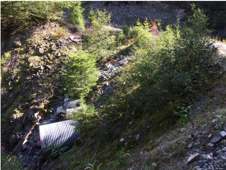
Fill over culverts
